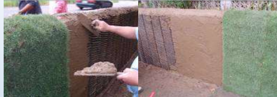
C. Coat Pipe Surface With Soil & Preplant In Nursery
