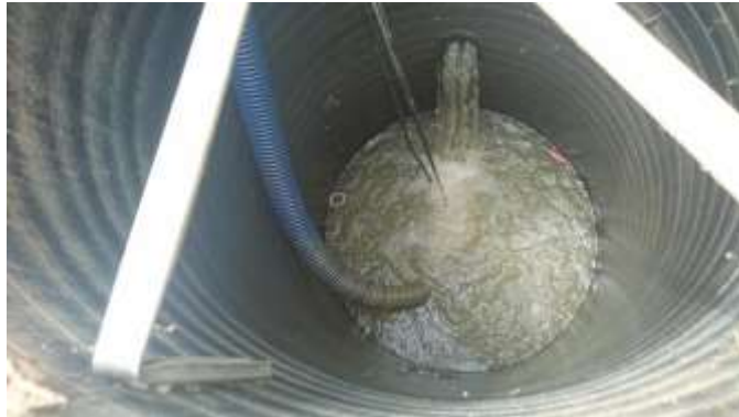
Pumping away groundwater to lower groundwater level
