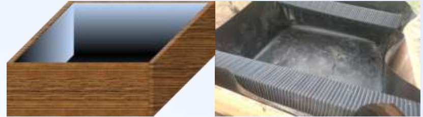
2. Cover water membrane inside the garden edges
