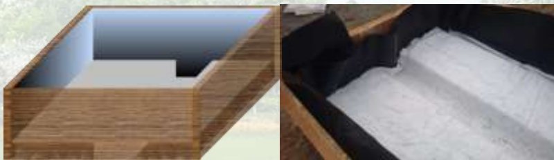
5. Lay textile fabric over mesh pipes
