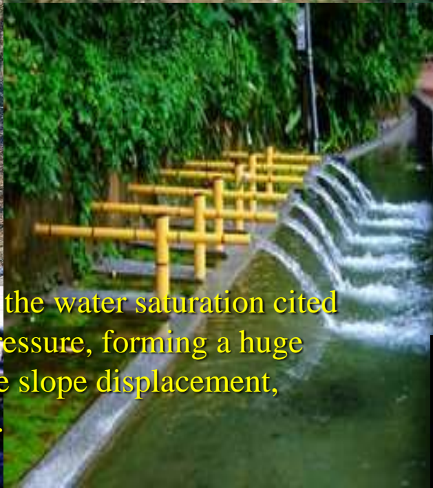
Mesh Drain pipe - Deep slope a certain depth, the water saturation cited unearthed in lower water pressure, forming a huge retaining wall to prevent the slope displacement, landslides and debris flows.
